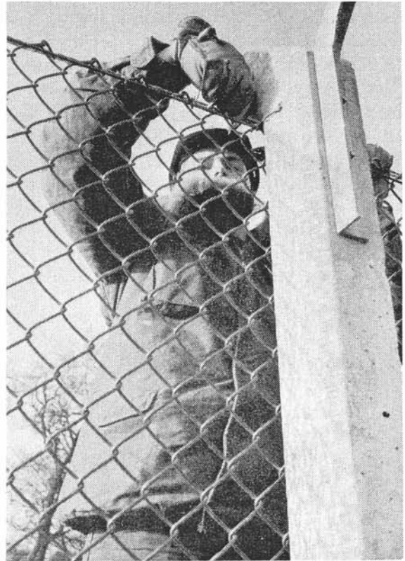
Finishing up: E03 Menning of Seabee Det 3, puts the final touches on the Base Perimeter Fence Project.
