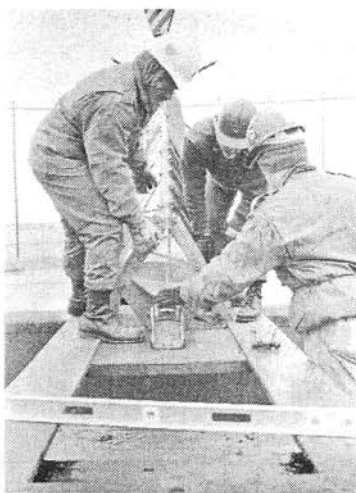
Antenna maintenance can be physically demanding...
