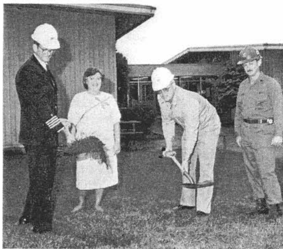
The Halsey School Lunchroom Project started by NMCB-40, 9 August 1989.
