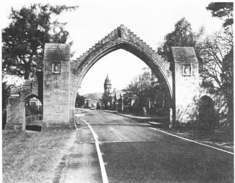
The Dalhousie Arch in Edzell Village where the base derives its name.
